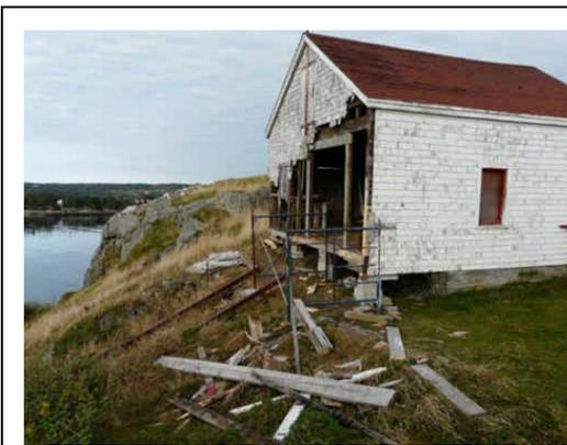
Boathouse south wall in the process of being repaired. Harsh weather and no maintenance in recent years left this building in jeopardy.
