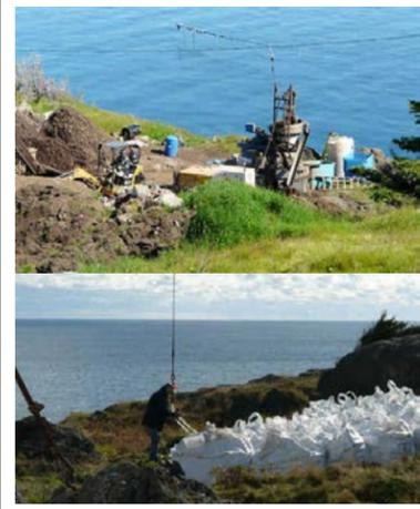
CleanEarth Technologies crew sieving lead paint contaminated soil at Swallowtail. Bags of contaminated soil were removed by helicopter.
